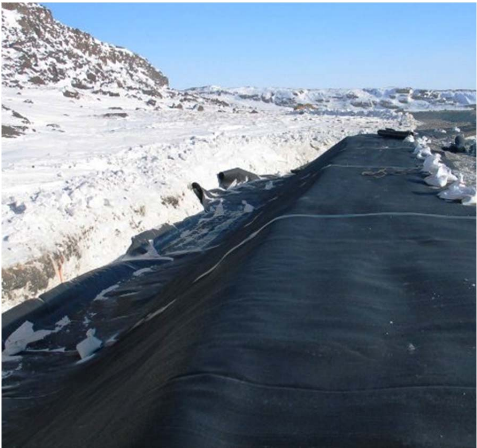
Photo 8: Layfield cleaning trench before liner installation Photo 9: HDPE Liner Stn 2+95 to 3+30
