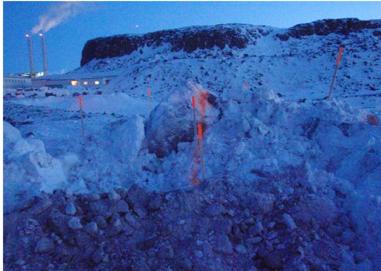
Photo 22: ~SW view of underbuilt US toe slope around station 1+20. A screenshot of the as-built isopach (from 2012/0313) is included to better highlight this slightly underbuilt area. This area is planned to be built up to grade in the coming days.
