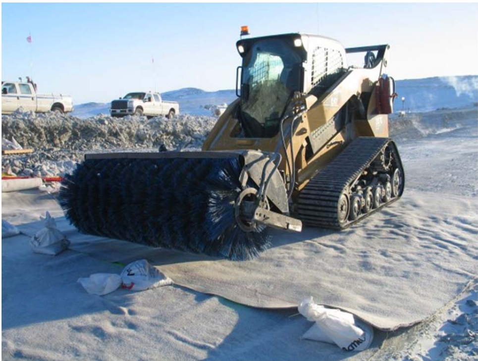
Photo 5 (left): Skid Steer was used to anchor the GCL Photo 6 (right): Set up. Skid Steer holding down GCL. Excavator pulling and unrolling the GCL.
