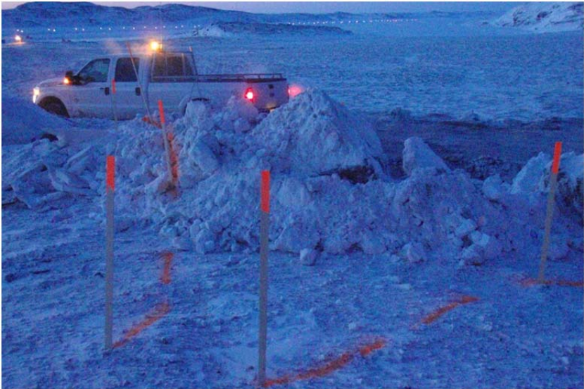
Photo 22: ~SW view of underbuilt US toe slope around station 1+20. A screenshot of the as-built isopach (from 2012/0313) is included to better highlight this slightly underbuilt area. This area is planned to be built up to grade in the coming days.
