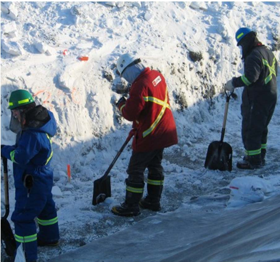
Photo 8: Layfield cleaning trench before liner installation Photo 9: HDPE Liner Stn 2+95 to 3+30
