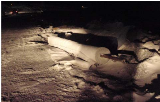
Photo 16 & 17: GCL rolls left outside at the DS dam shell and by the FCP hopper
