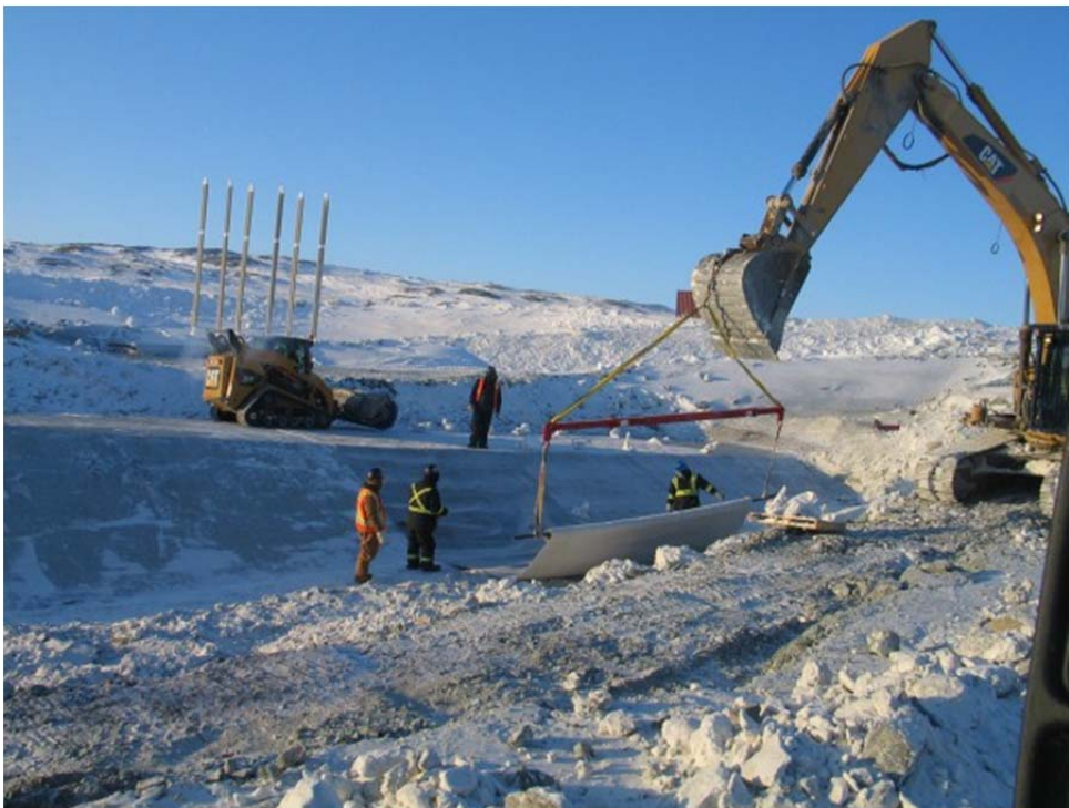
Photo 5 (left): Skid Steer was used to anchor the GCL Photo 6 (right): Set up. Skid Steer holding down GCL. Excavator pulling and unrolling the GCL.
