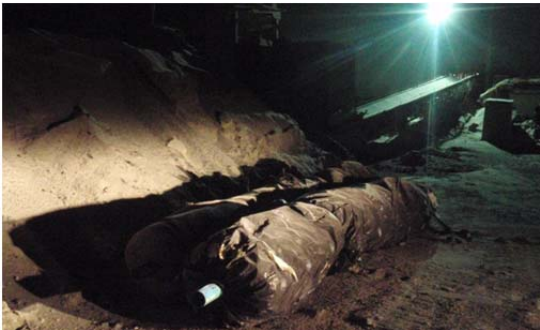
Photo 16 & 17: GCL rolls left outside at the DS dam shell and by the FCP hopper
