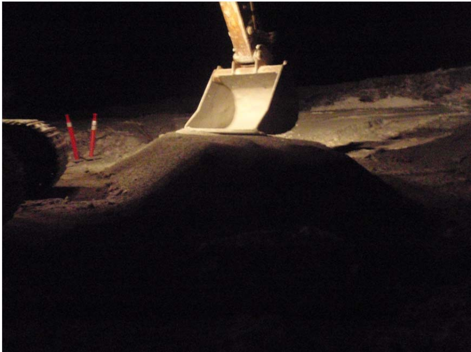
Photo 20 and 21: ~ ESE and SW view respectively of the 330 excavator spreading crush over multibead cables at 0+40.
