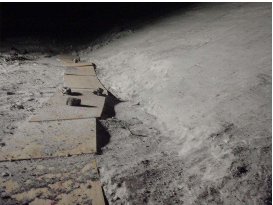
Photo 22: ~SW view of underbuilt US toe slope around station 1+20. A screenshot of the as-built isopach (from 2012/0313) is included to better highlight this slightly underbuilt area. This area is planned to be built up to grade in the coming days.
