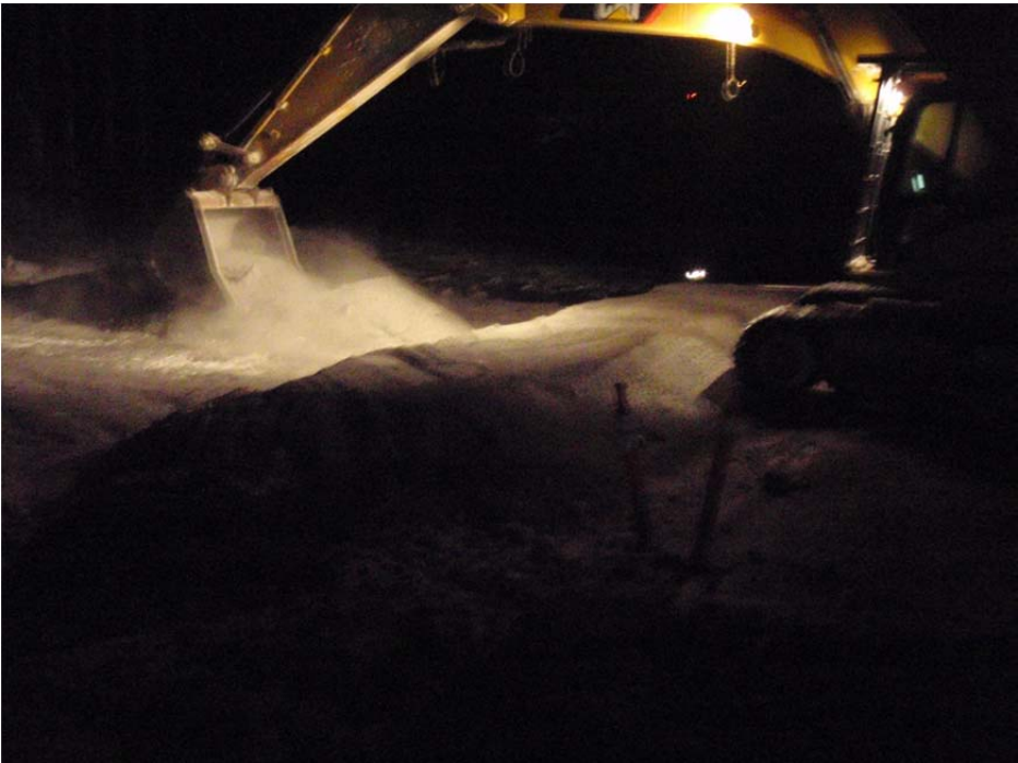
Photo 20 and 21: ~ ESE and SW view respectively of the 330 excavator spreading crush over multibead cables at 0+40.
