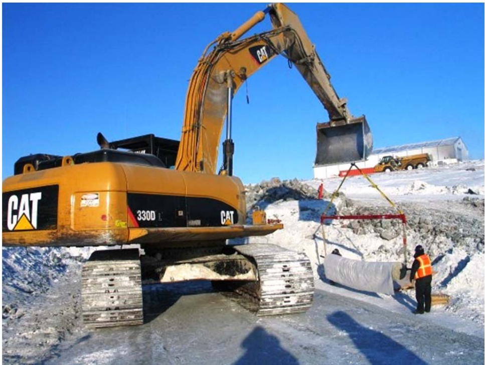
Photo 4 (right): Excavator was used to handle GCL roll. In this photo it is on top. In the end it was positioned at the bottom.
