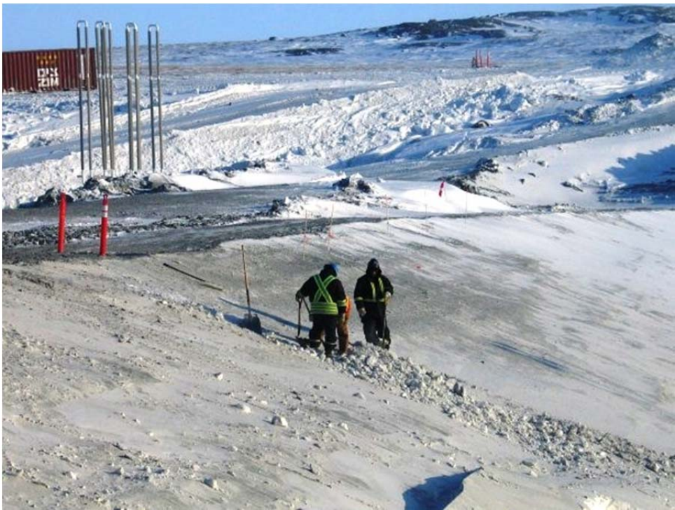
Photo 3 (left): Labourers cleaning core slope by hand.
