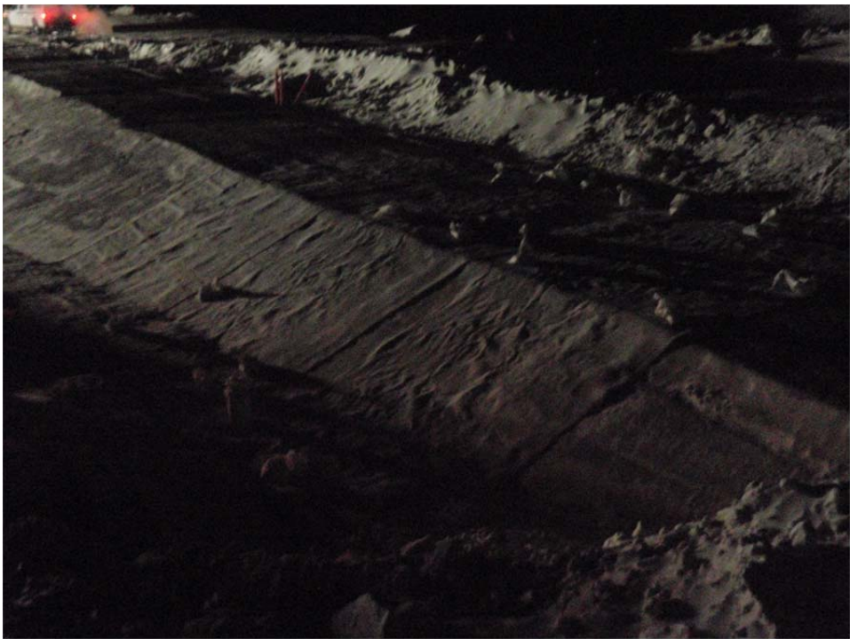
Photo 14: View of three 'trial' GCL panels placed on dayshift.
